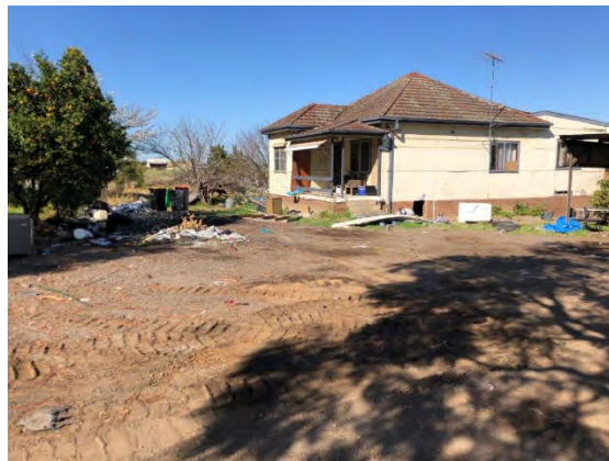
TP201 – fibre cement building located in the vicinity of TP201
