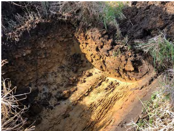
TP207 – typical subsurface conditions comprising reworked sandy clay overlying natural clay
