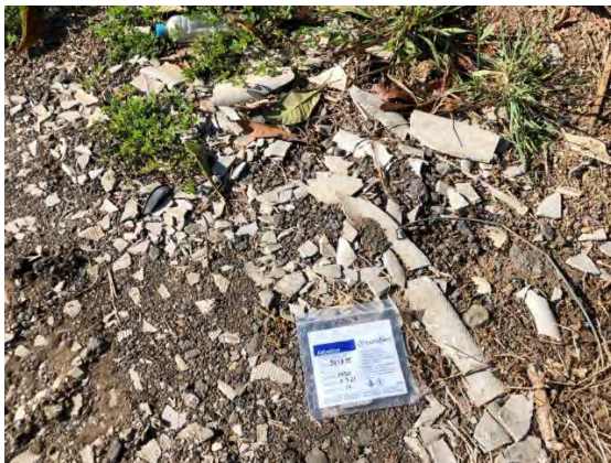
MS01 – asbestos debris located on the surface of the driveway
