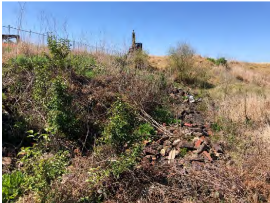
Area near TP07 – embankment consisting of building demolition waste, north-easterly aspect
